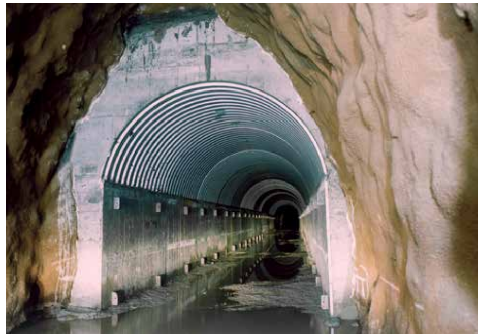
Fig. 18. The tunnel from Lake Päijänne was repaired for the first time in 1999. The reinforcement method used here is an exception and only used in cases of severe collapse. Some parts were bolted and shotcreted while most parts are still without any reinforcement. (Photo: Foto Mannelin Oy)
