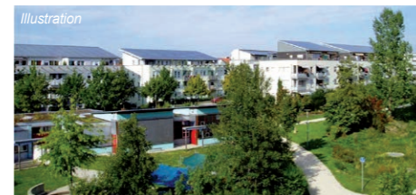
Several solar panels installed on the roofs of buildings and connected directly to the network: estimated surface area 10 m² /lodging.
